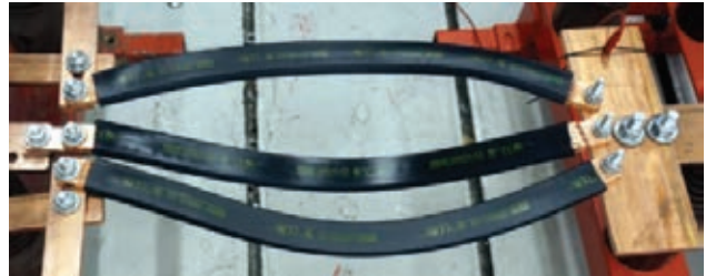
After Short-circuit test
